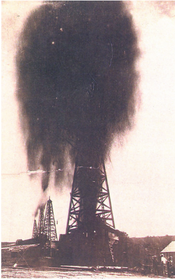
Oklahoma oil well blowout
